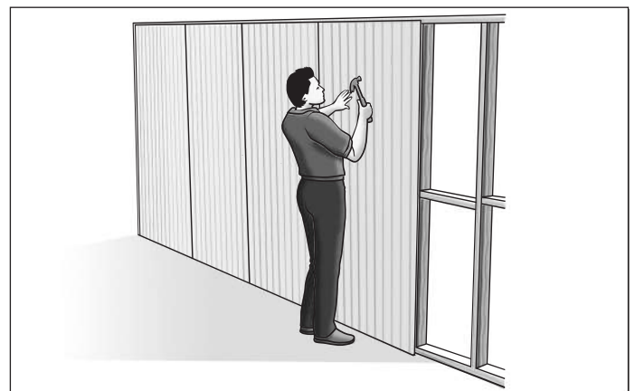
FIGURE 5 SHEET FIXING
