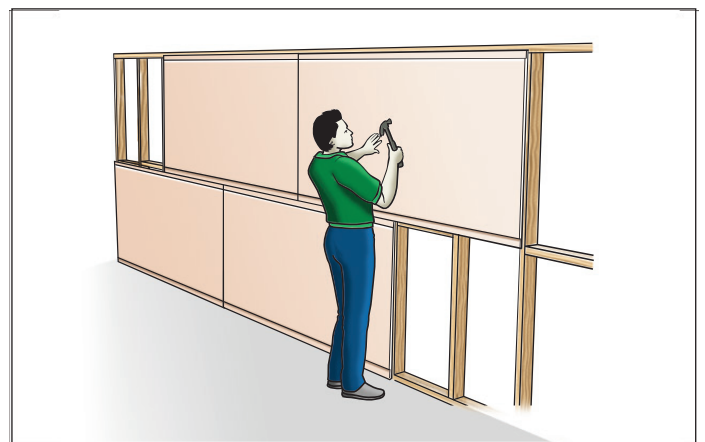
FIGURE 5 FIXING REMAINING SHEETS
