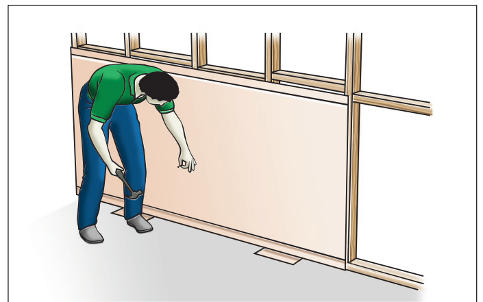
FIGURE 4 FIXING FIRST SHEET
