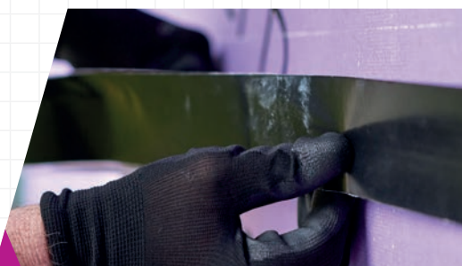
Weather Defence Joint Tape being applied
