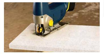
This is applicable for panels up to 25mm thick. The panels can be cut easily with a jigsaw to form various shapes. Blades with special hardened teeth are available for cutting PROMATECT® 100 boards. As with all power tools, care should be taken to cut within the capacity of the tool and blade. Do not force the cutting speed.
