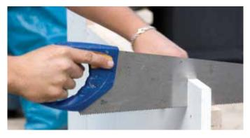
Hand sawing is suitable for general cutting operations and for small cuts, notchings or small penetrations. However, this method of cutting can be rather time intensive. The fastest way is to allow the saw to work at its own speed, trying to force the tool to cut faster merely blunts the teeth.
