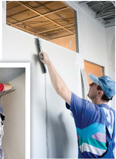
Plastering the board joints in partitions (above) and the junctions of wall and ceiling (left).
